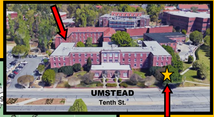
Dean of Students Office Handicap Accessibility Entrance
